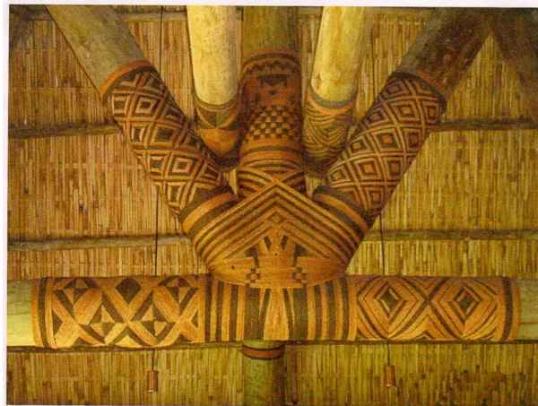
Figure 7 Black and Natural coloured 'afa used to bind cross-sectional piece in Samoan fale
